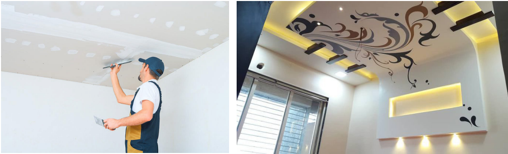
Fig. 1.2.19 False ceiling and drywall installer engaged in false ceiling work
