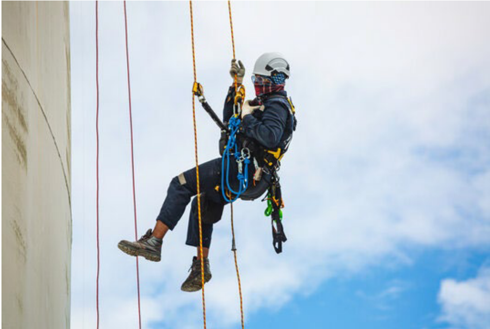
Fig. 1.2.12 Safety during work
