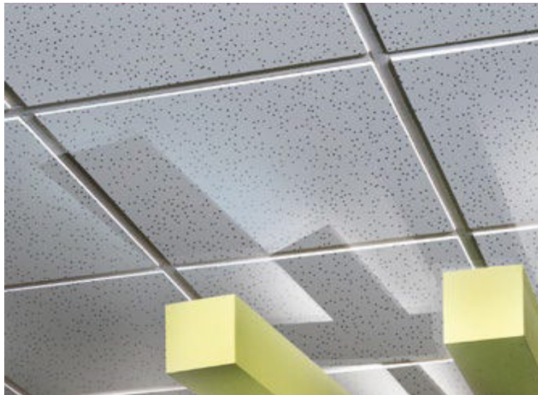
Fig. 5.1.1: Exposed grid suspended panel ceiling system
