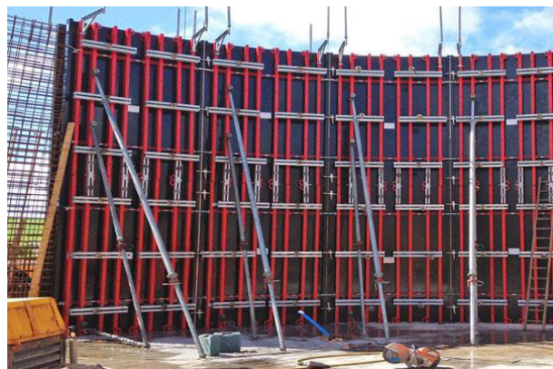
Fig. 1.1.14 System formwork
