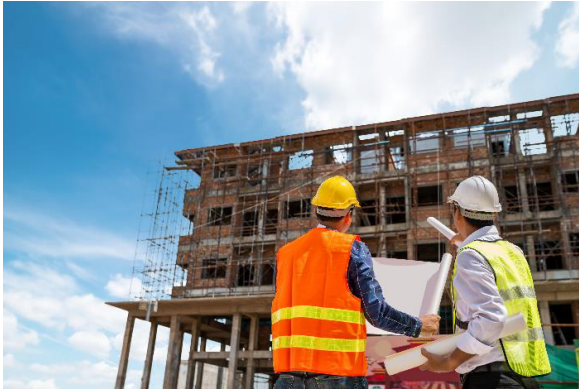
Fig. 1.1.4 Building Construction Site
