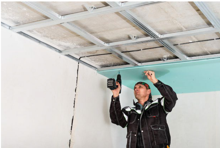
Fig. 4.1.35: Check spacing and alignment
