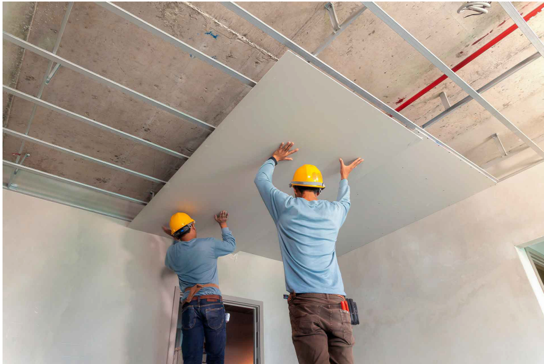
Fig. 3.2.20: Fixing the perimeter in false ceiling and drywall installation
