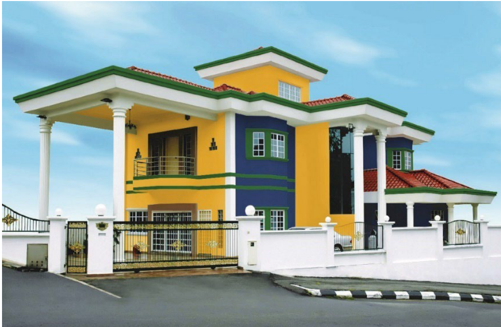
Fig. 1.2.10 Exterior painting and coating
