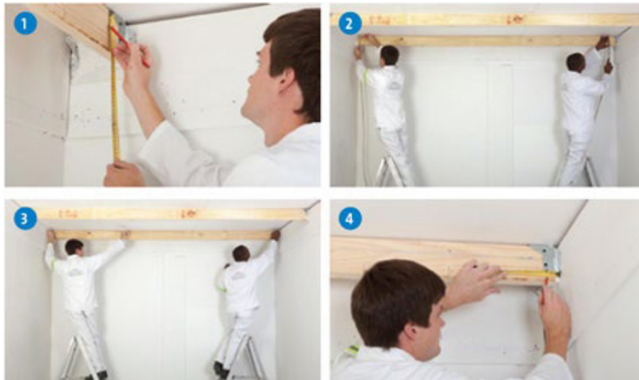
Fig. 5.2.7: Fixed flush jointed ceiling installation
