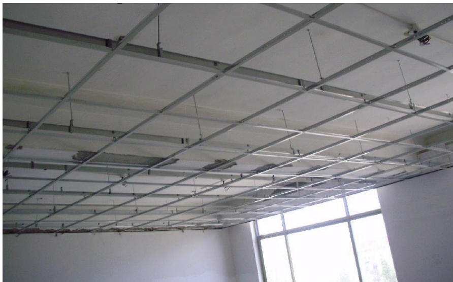
Fig. 4.2.19: Finishing the installation of a suspended flush jointed ceiling system
