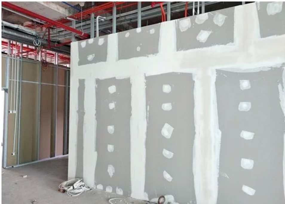
Fig. 6.1.16: Dry fit the panels in their intended positions
