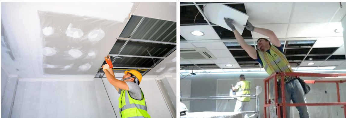
Fig. 1.2.17 False ceiling and dry wall installer
