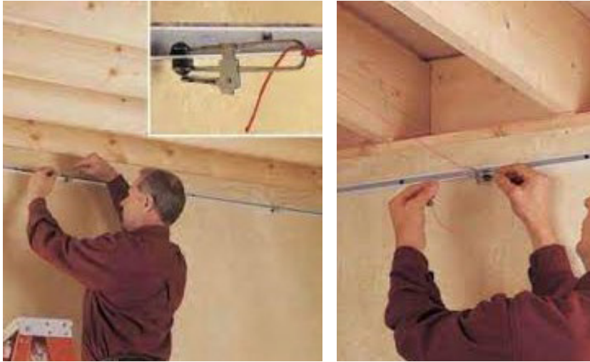
Fig. 3.3.17: Mark the location of ceiling brackets
