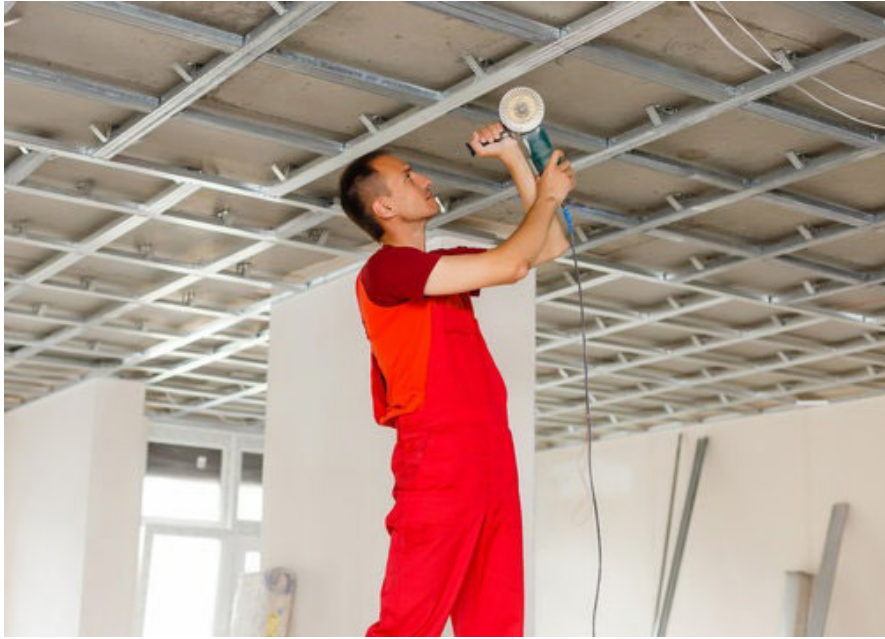
Fig. 4.1.34: Position the framing system
