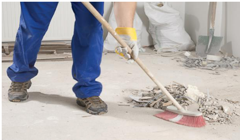
Fig. 9.3.5 Clean-up Debris and Waste
