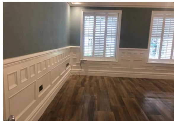
Fig. 6.1.6: Installation of wall panels
