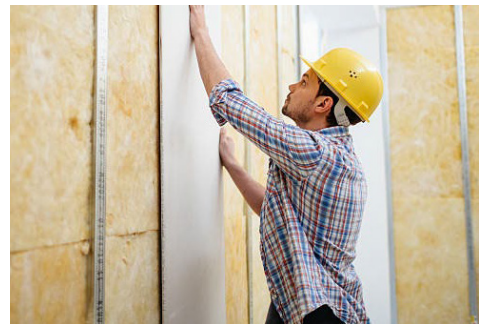
Fig. 4.1.38: Plasterboard placement
