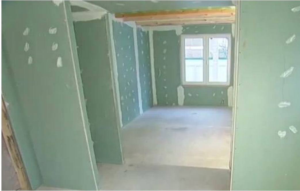
Fig. 6.2.10: Finishing of panel joints as per instructions
