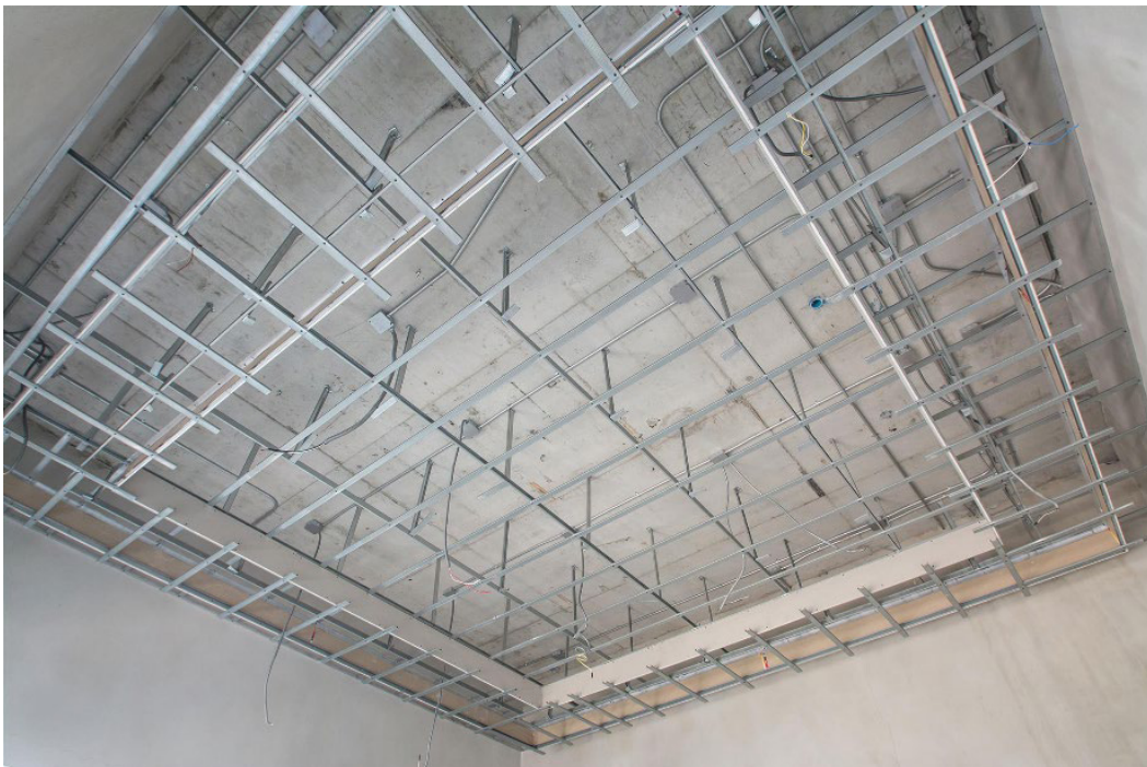
Fig. 3.2.22: Accurate placement and alignment of the ceiling framework
