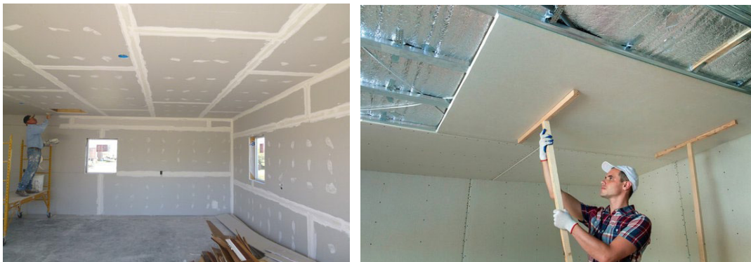
Fig. 6.2.1: Installation of ceiling and wall frames
