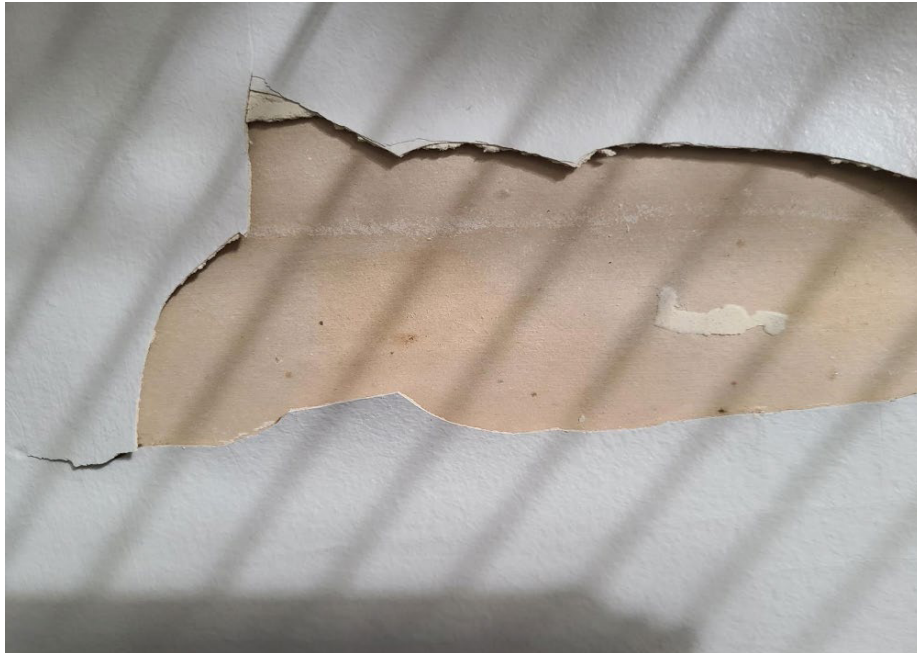
Fig. 4.2.18: Inspect for defects
