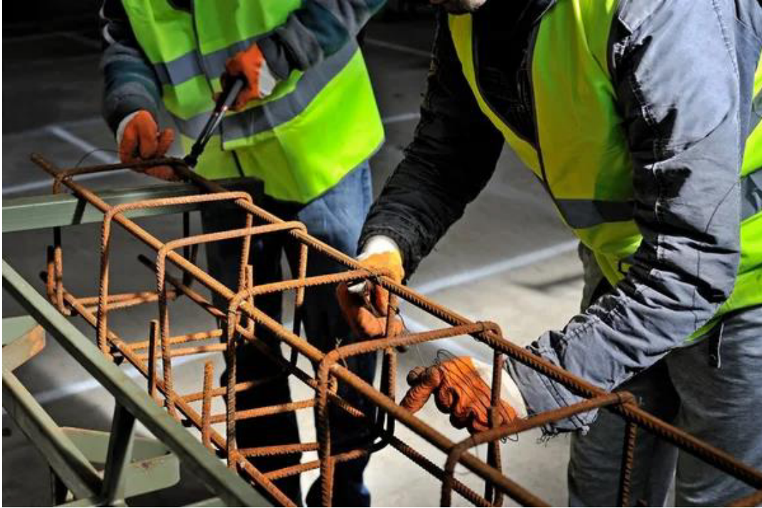
Fig. 8.2.4 Effectively collect and dispose of waste generated during bar bending activities
