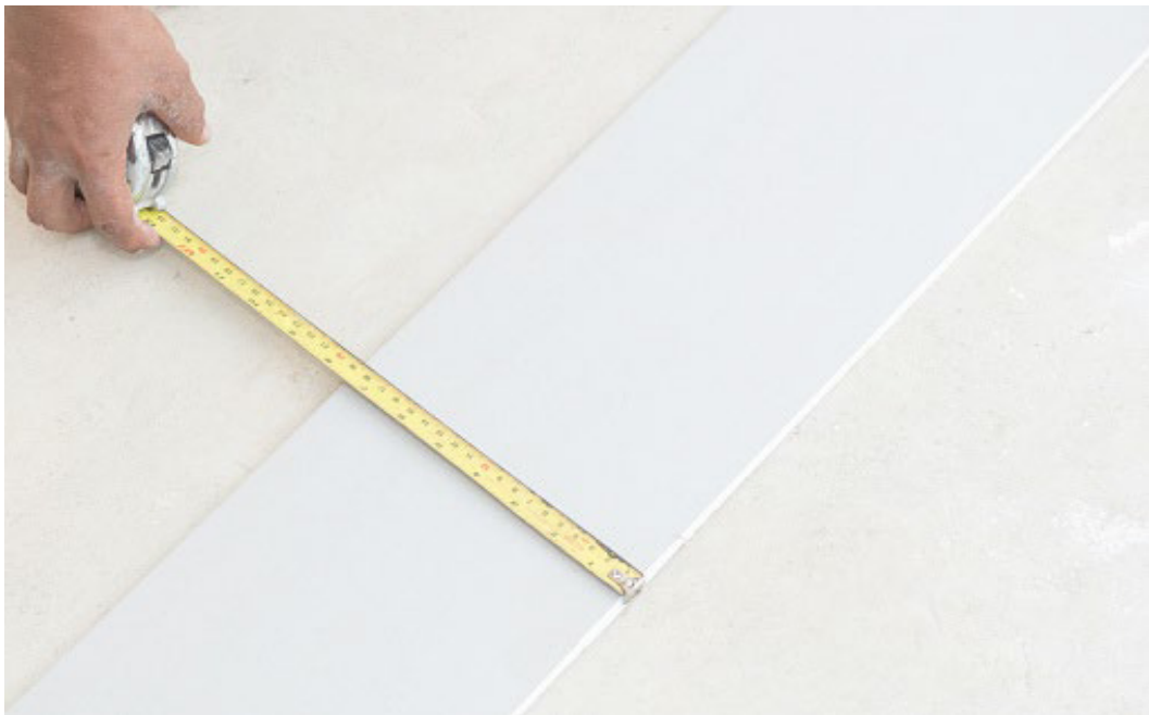
Fig. 3.3.5: Make sure of boards are measured accurately
