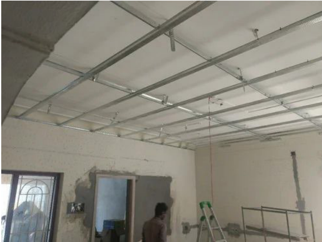
Fig. 3.3.10: Starting and end point of false ceiling installation
