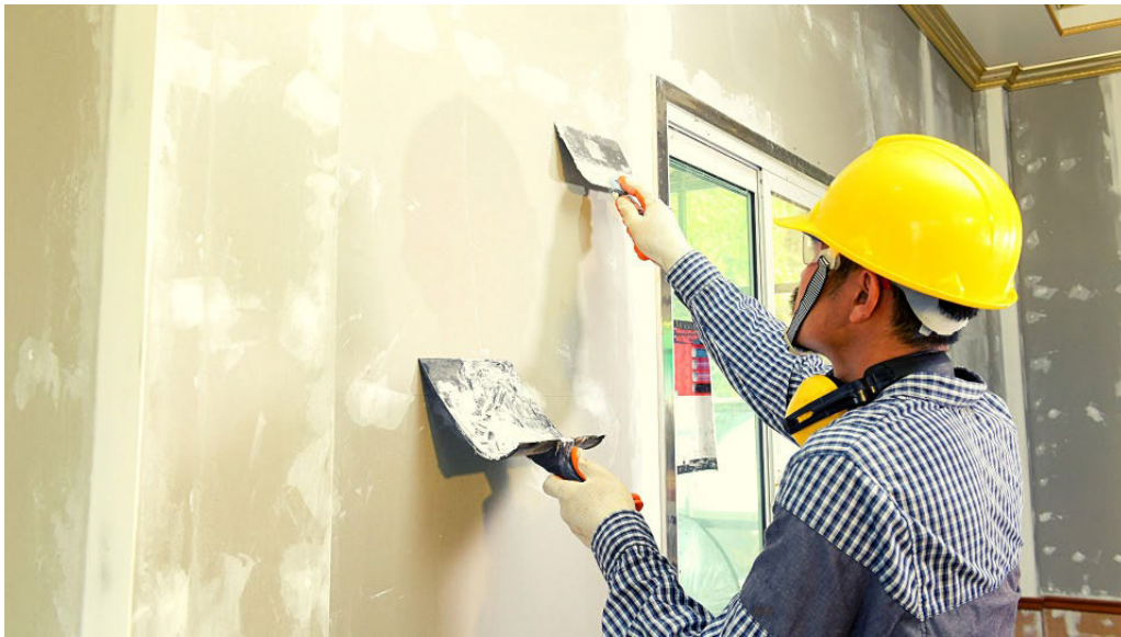
Fig. 1.2.2 Drywall and plastering
