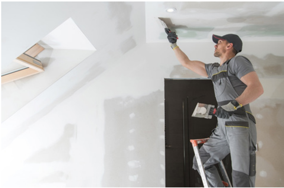
Fig. 5.2.32: Effectively covering and finishing joints and edges of plasterboard panels
