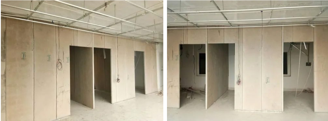
Fig. 6.2.2: Vertical frame and joints in the frames
