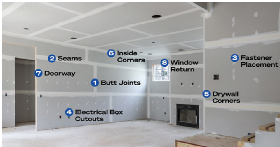
Fig. 6.2.8: Fixing of horizontal and vertical panels
