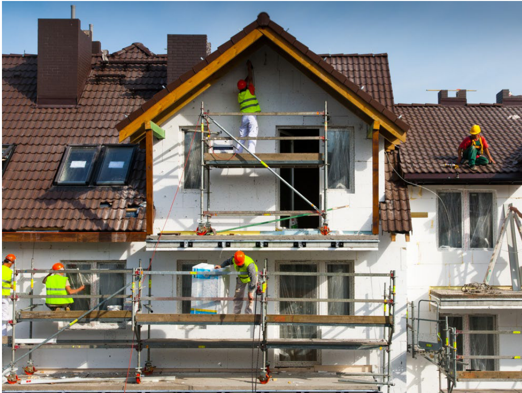
Fig. 1.2.20 Work related to exterior finishes
