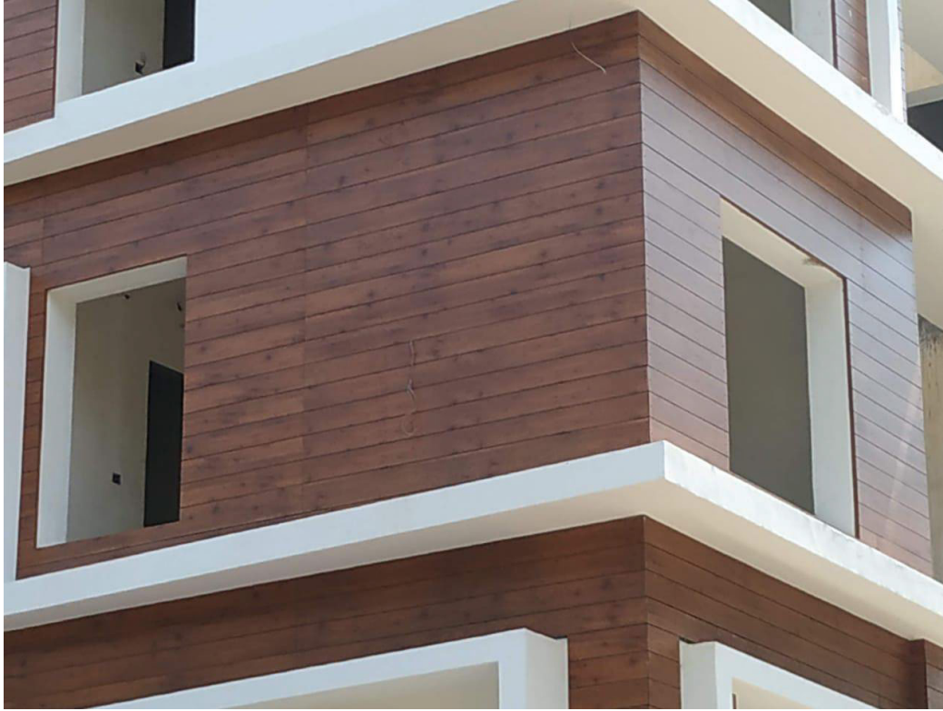
Fig. 1.2.8 Exterior cladding
