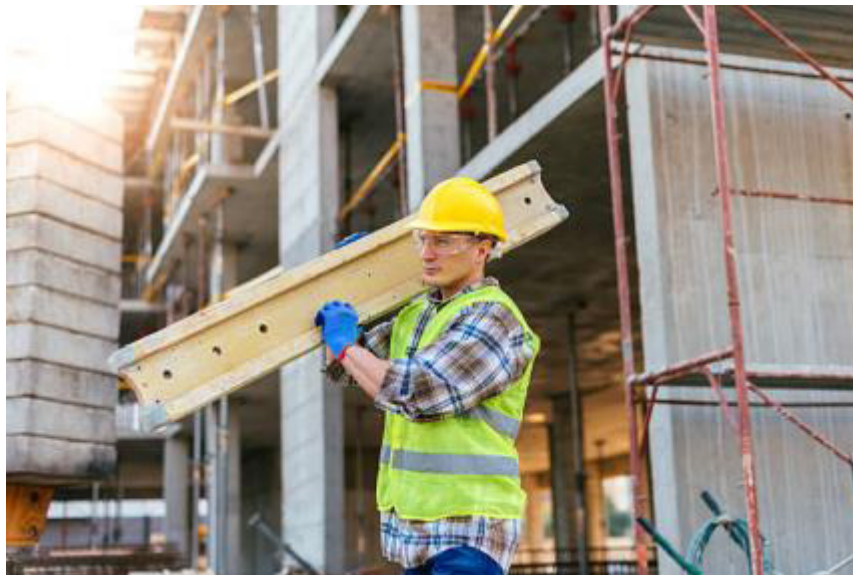
Fig. 9.3.11 Material Handling with Safety
