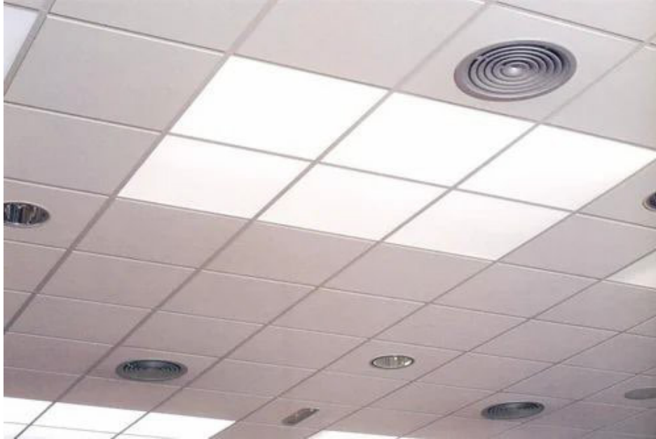
Fig. 5.1.6: Providing cut-outs using appropriate tools
