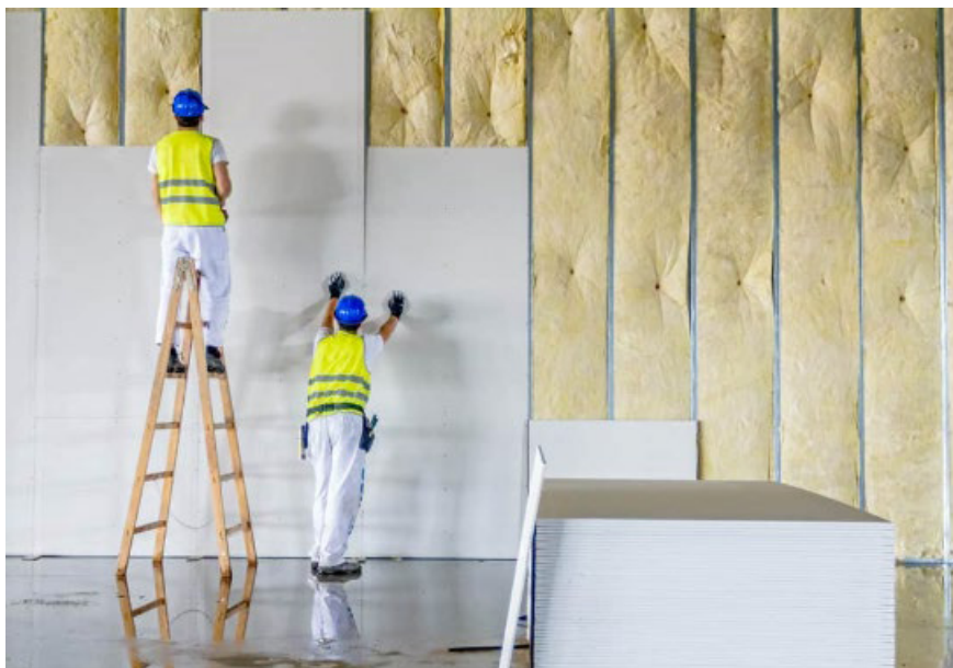
Fig. 6.1.1: Dry wall installation
