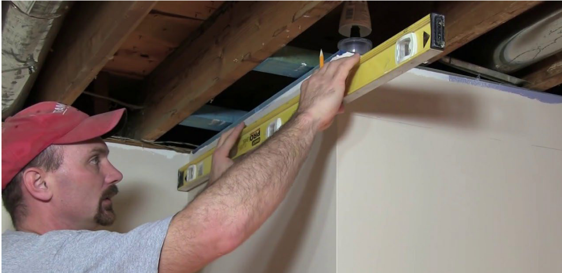
Fig. 3.2.19: Using levelling tools
