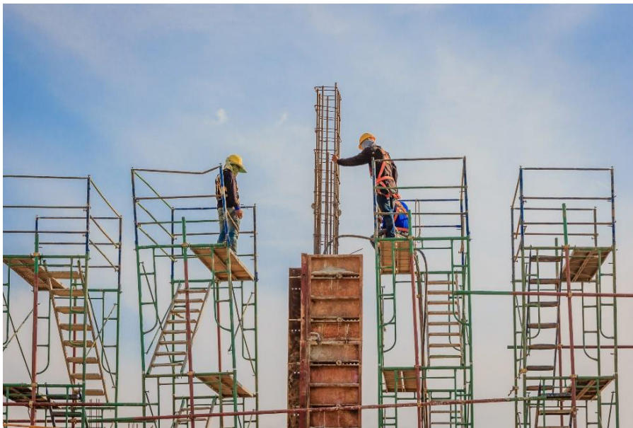
Fig. 7 .1.4 Coordination during Construction Work
