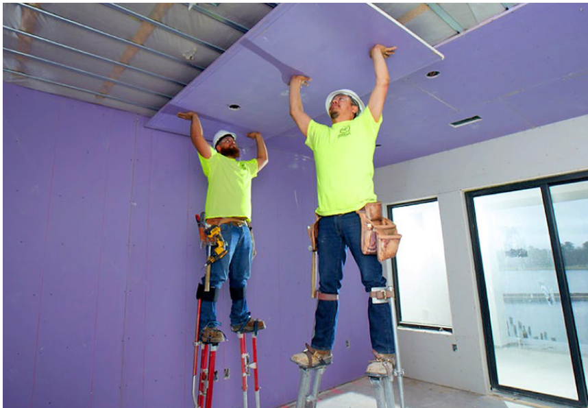
Fig. 4.1.33: Installation of a non-suspended flush jointed ceiling system
