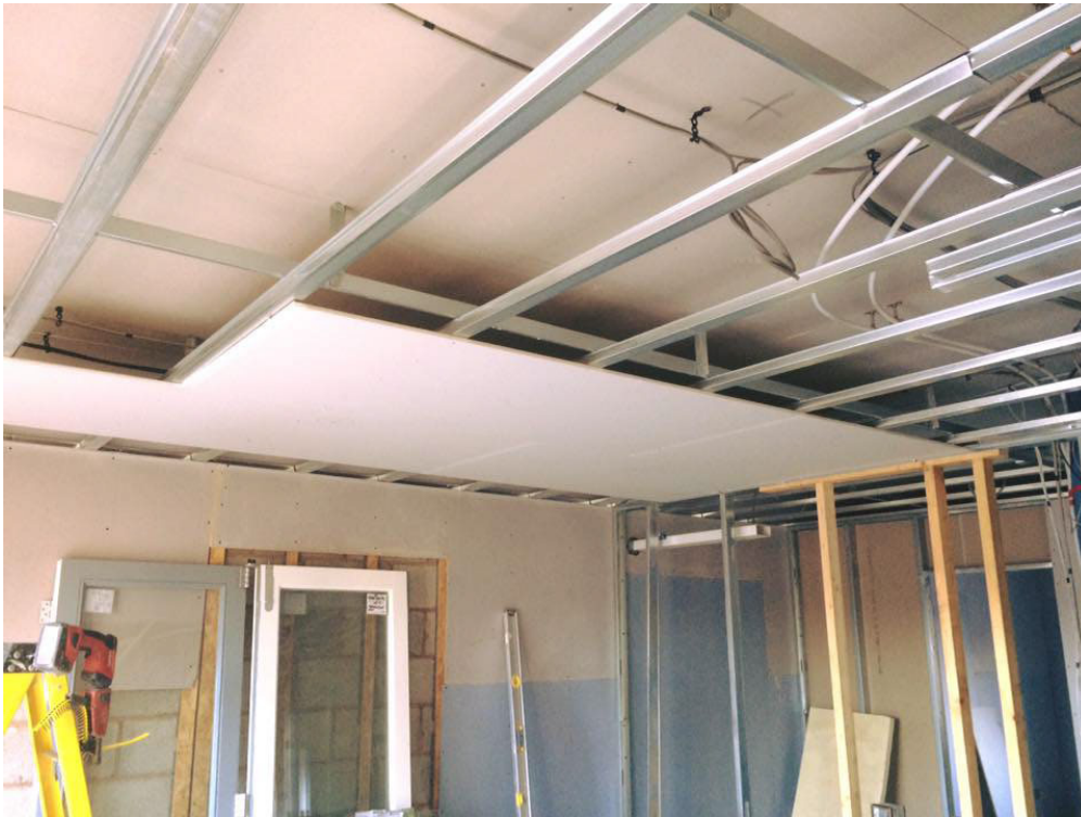
Fig. 4.1.31: Process of measuring and marking the correct height and alignment
