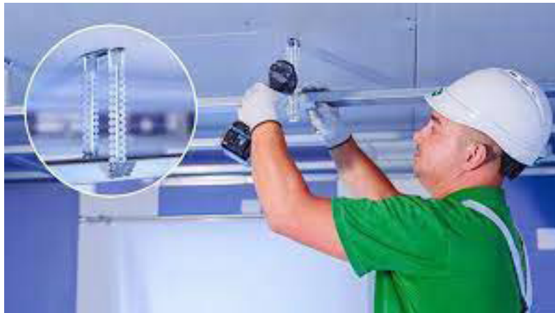
Fig. 5.2.12: Bracket installation
