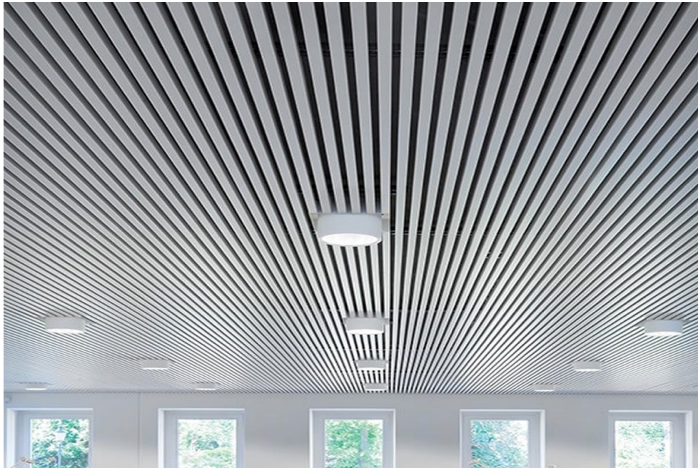
Fig. 5.1.7: Installation of fixtures
