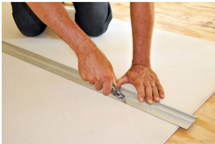
Fig. 5.2.17: Marking and cutting of the plasterboard as per the required shape
