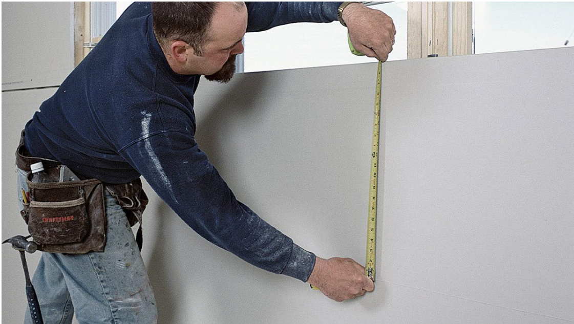
Fig. 6.1.15: Measuring the wall
