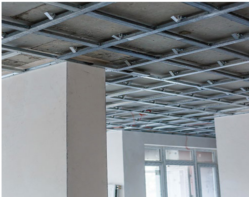
Fig. 4.1.32: Marking the perimeter
