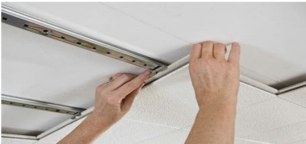
Fig. 4.1.28: Installing ceiling panels
