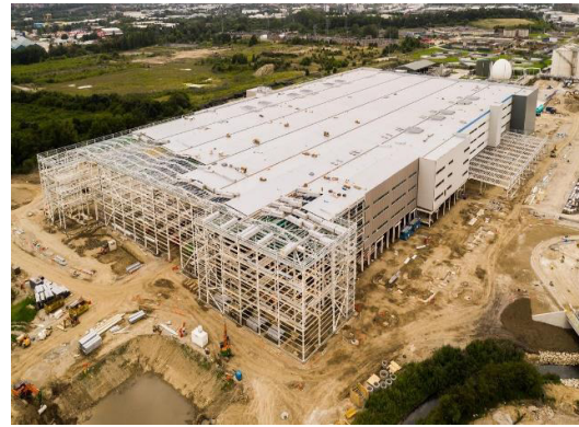
Fig. 1.1.5 Industrial Building Construction Site
