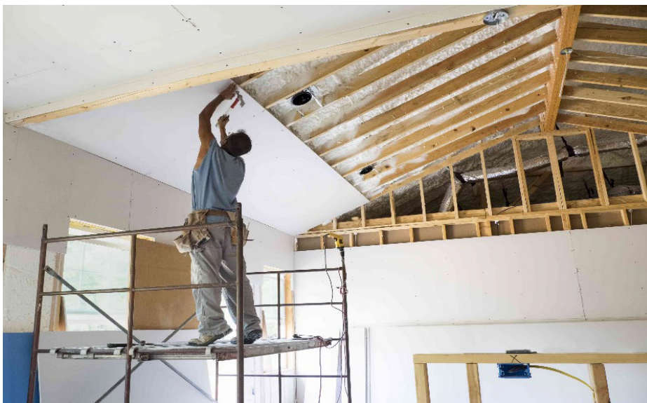
Fig. 4.2.17: Fixing of plasterboards to the Ceiling Sections
