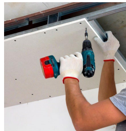
Fig. 3.2.12: Fasten the gypsum board
