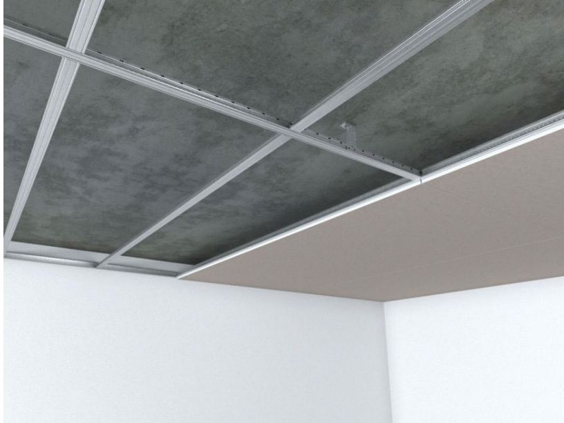
Fig. 4.1.20: Non-suspended flush jointed ceiling system
