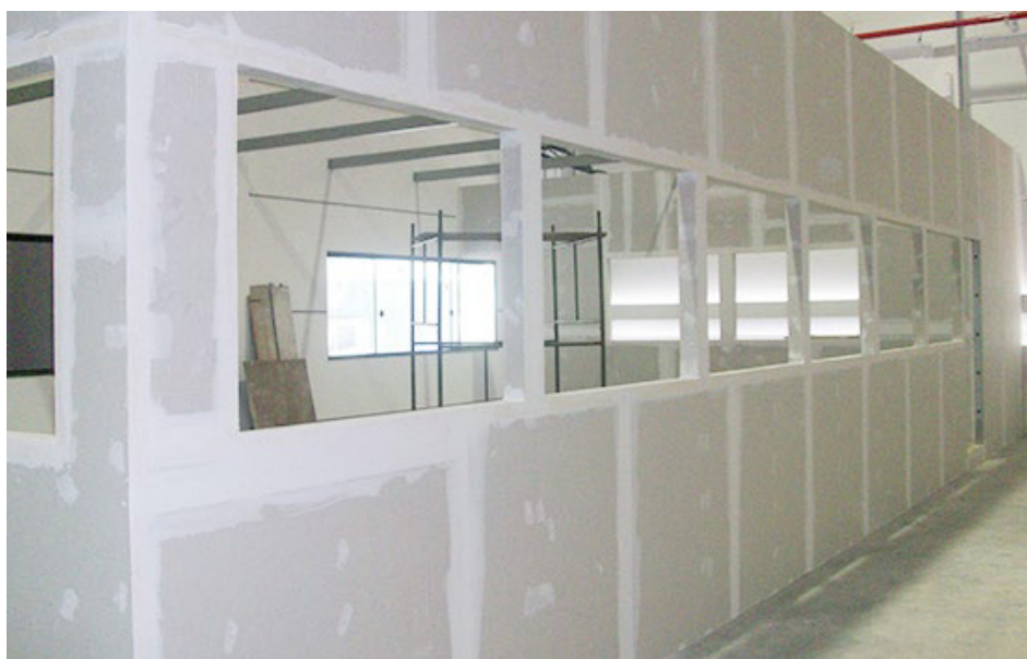
Fig. 6.2.4: Ensuring boards are accurately marked and cut
