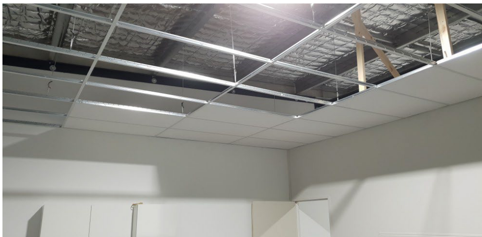
Fig. 5.2.6: Suspended ceiling installation
