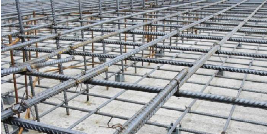
Fig. 1.1.12 Reinforcement bars fixed at site
