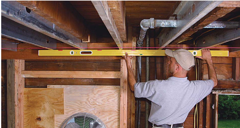
Fig. 3.3.13: Confirm heights or levels
