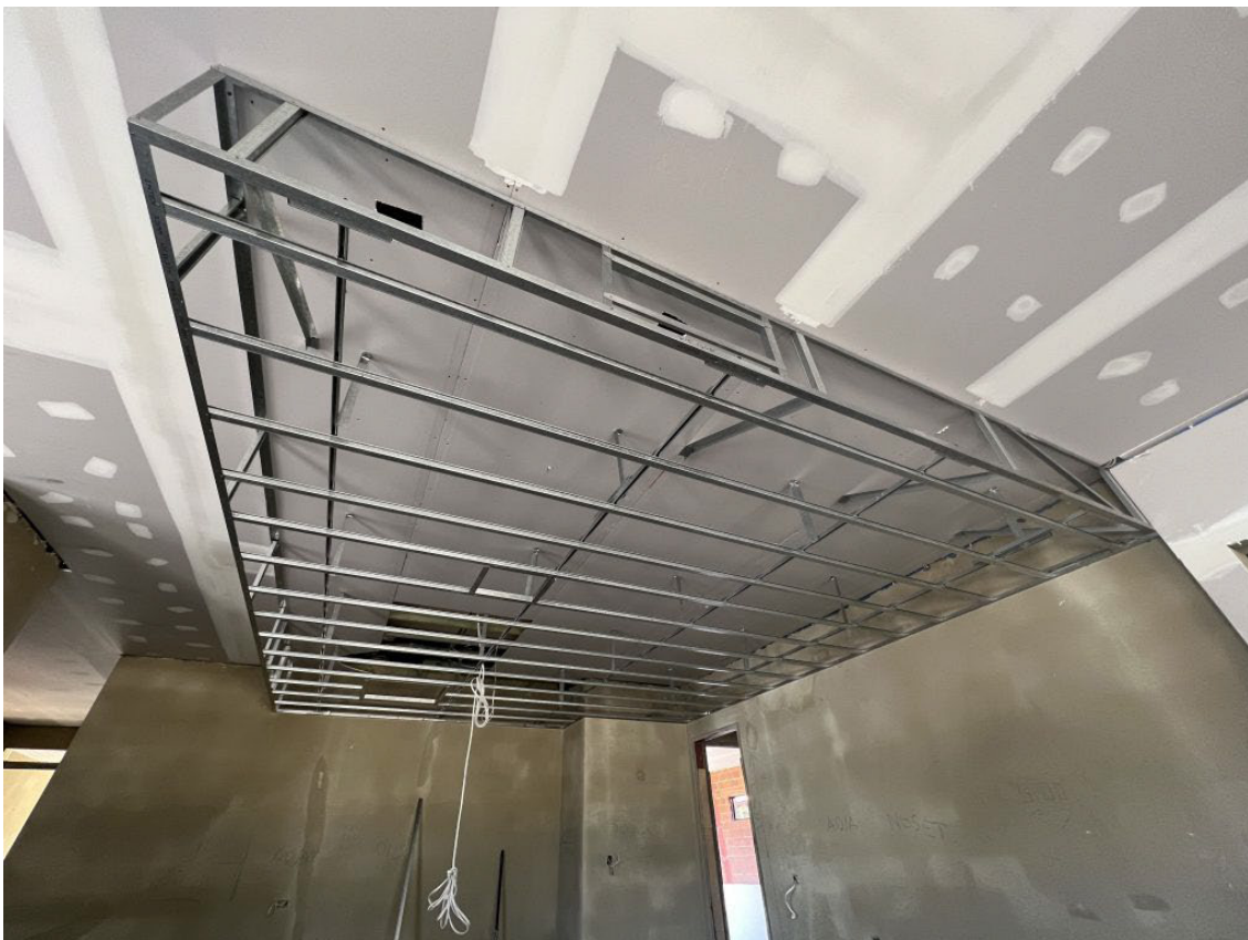
Fig. 3.3.3: Check the clearance for carrying out the false ceiling work
