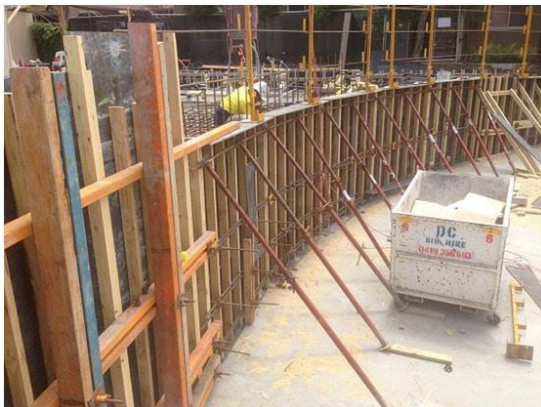
Fig. 1.1.13 Conventional formwork
