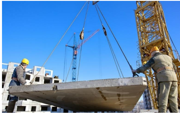
Fig. 1.1.17 Rigging work at site
