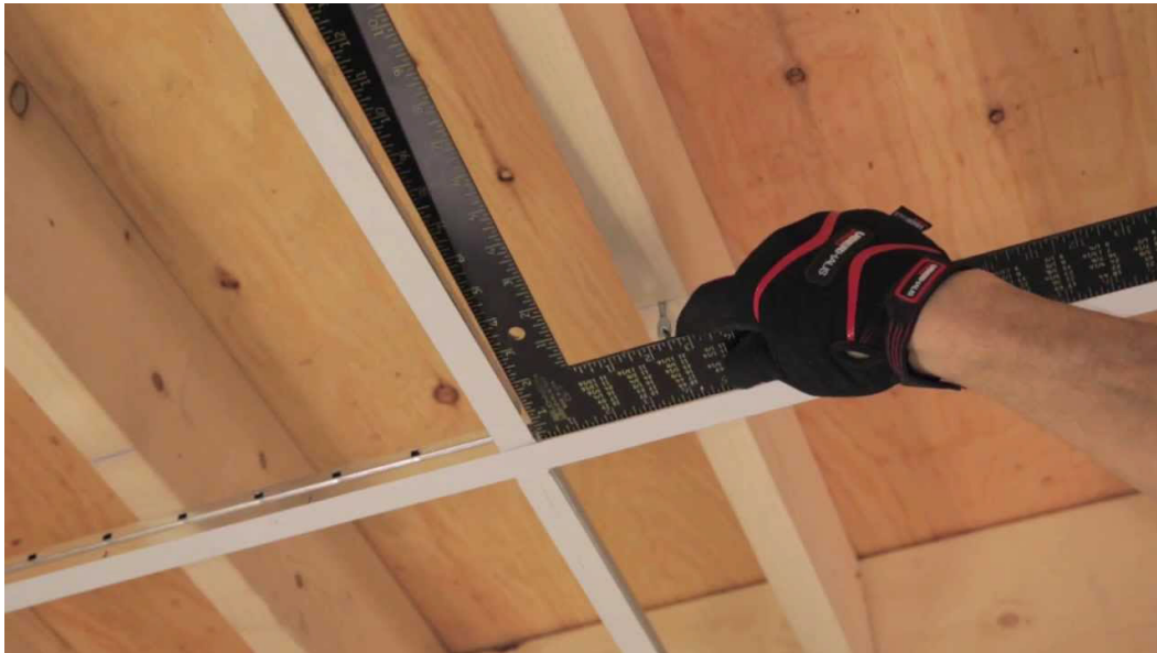
Fig. 3.2.26: Levelling and marking tools
