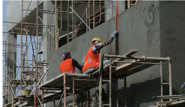
Fig. 1.1.10 Plastering Work
