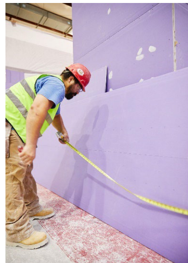
Fig. 4.1.42: Inspect the cut-out for any rough edges or imperfections
