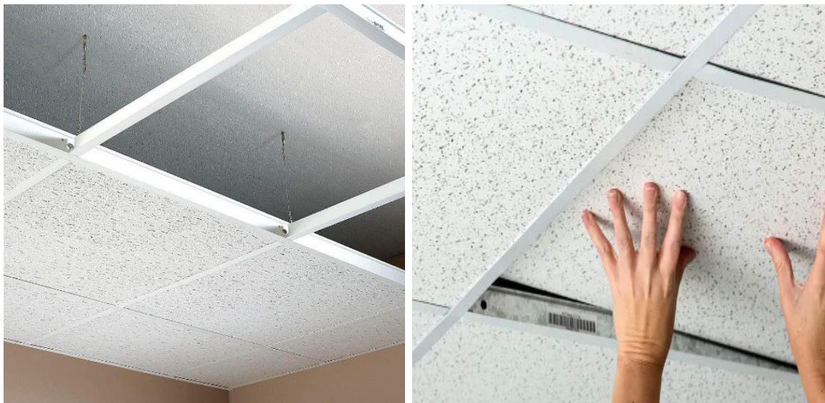
Fig. 4.2.3: Suspended flush jointed ceiling systems
