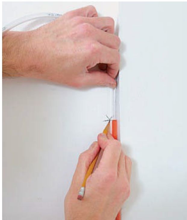
Fig. 3.3.16: Transfer the specified levels on the wall
