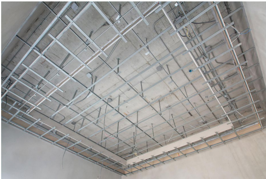
Fig. 4.2.16: Fixing and fitting of the ceiling sections
