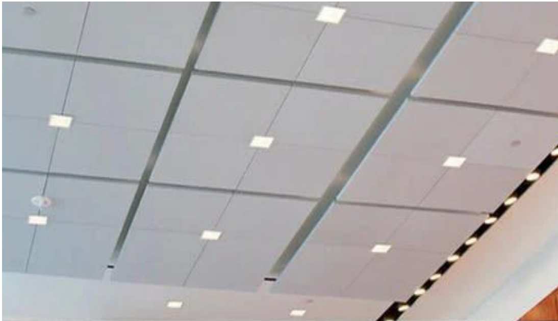
Fig. 1.2.7 Acoustic ceiling installation
