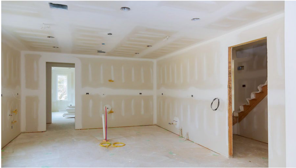
Fig. 1.2.15 Drywall installation
