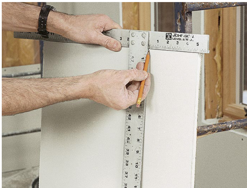
Fig. 4.1.29: Process of marking and cutting plasterboard
