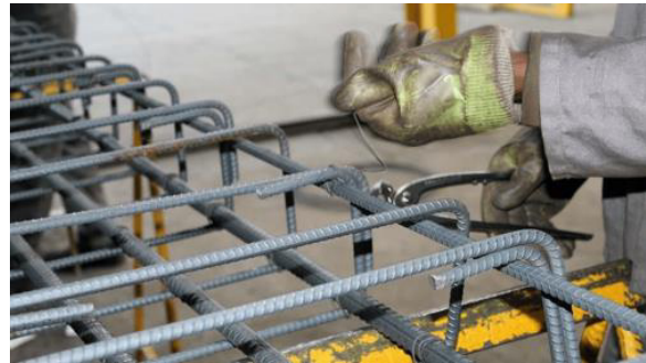
Fig. 1.2.1 Bar bending & steel fixing
