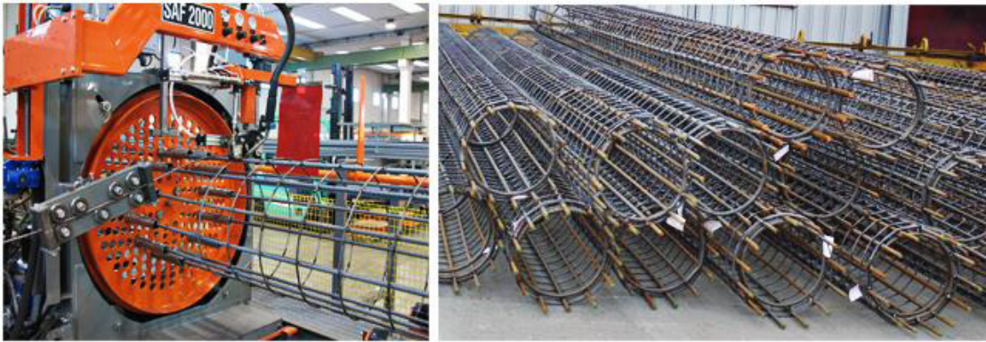
Fig. 5.3.8 On-site fabrication of a steel cage for reinforcing concrete structures
