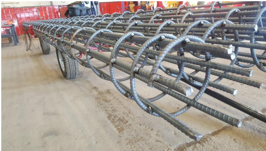
Fig. 5.2.3 RCC Cage Fabrication in various Structures
