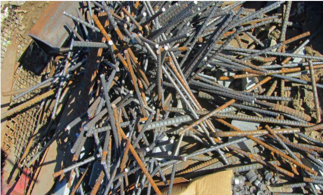
Fig. 8.2.4 Effectively collect and dispose of waste generated during bar bending activities
