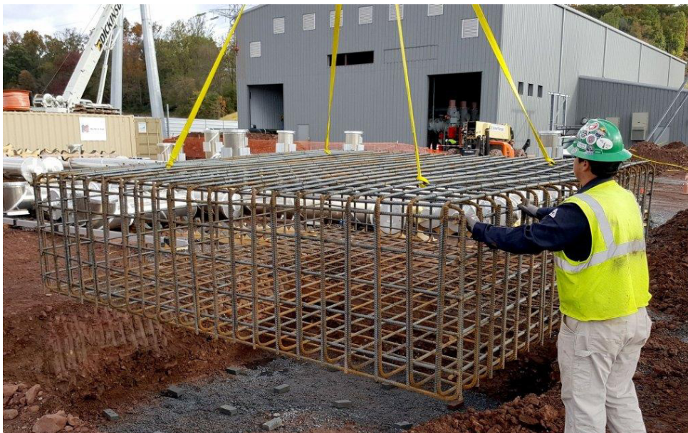
Fig. 5.3.6 Prefabricated cages
