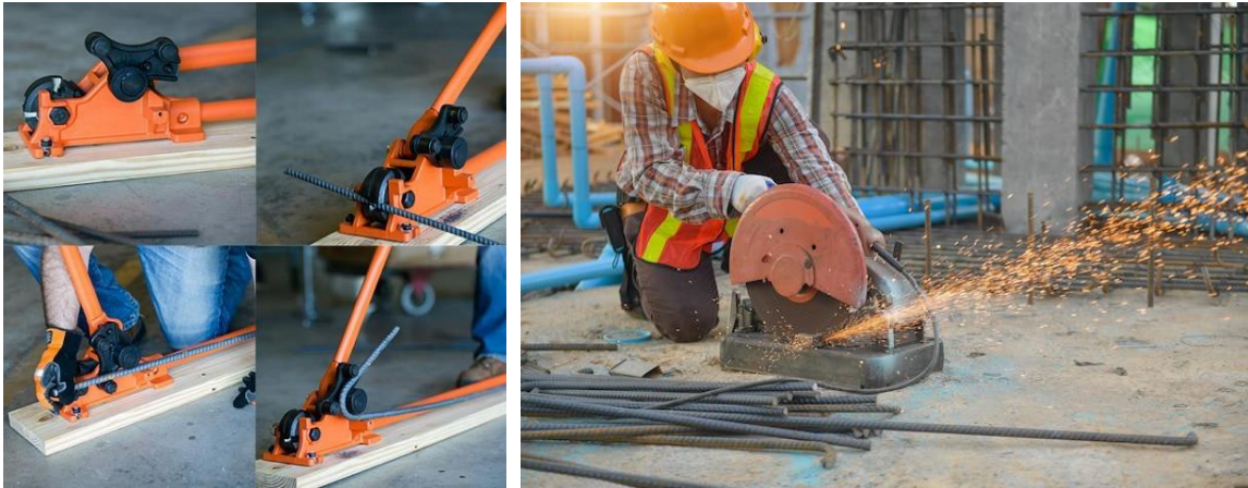
Fig. 1.2.5 Cutting of rebars
