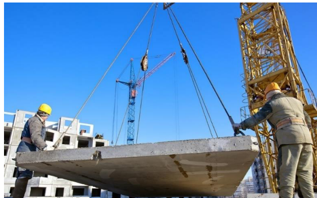
Fig. 1.1.17 Rigging work at site
