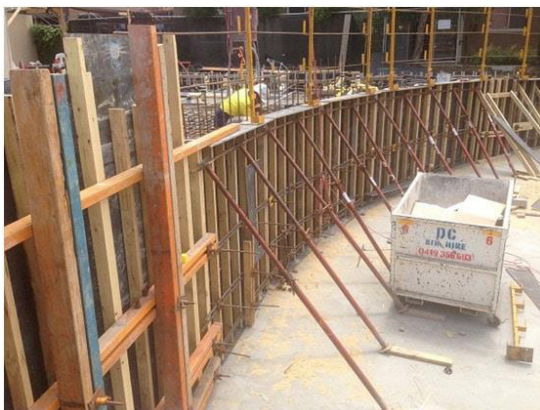
Fig. 1.1.13 Conventional formwork
