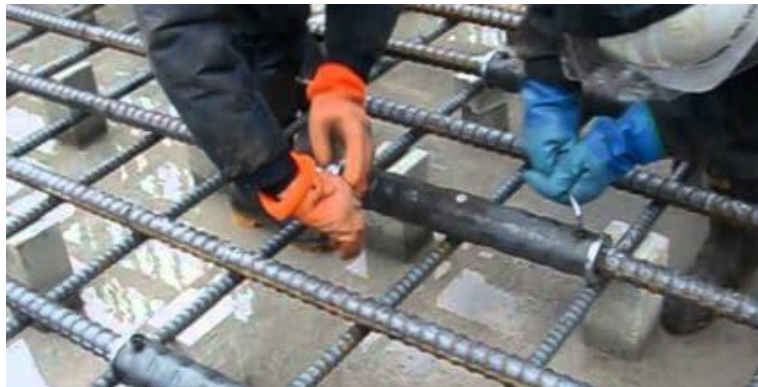
Fig. 5.1.4 Rebar splicing
