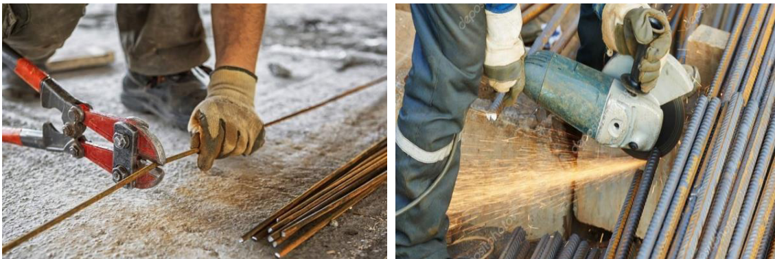
Fig. 4.3.20: Cutting preparation
