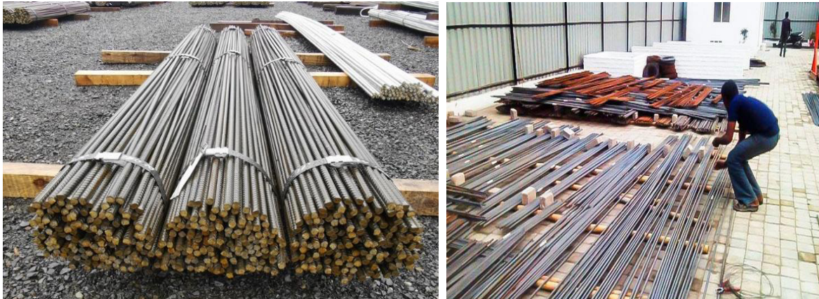
Fig. 4.4.4: Storage and stacking of rebars
