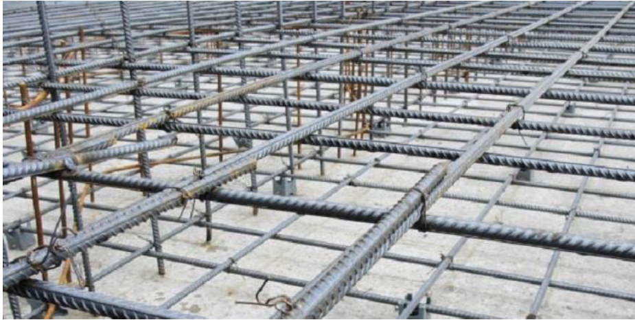
Fig. 1.1.12 Reinforcement bars fixed at site
