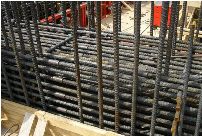
Fig. 5.1.7 Mechanical splicing
