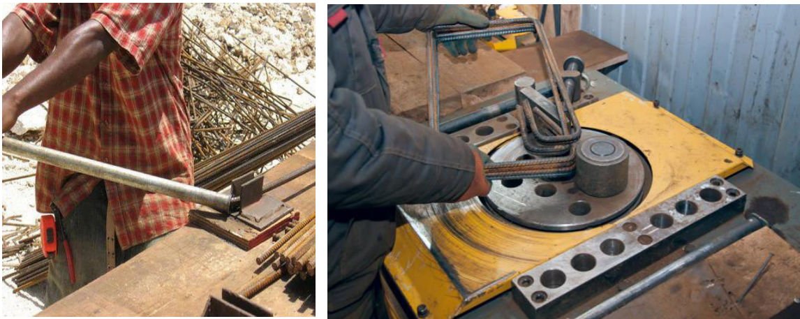
Fig. 1.2.6 Bending of a rebar
