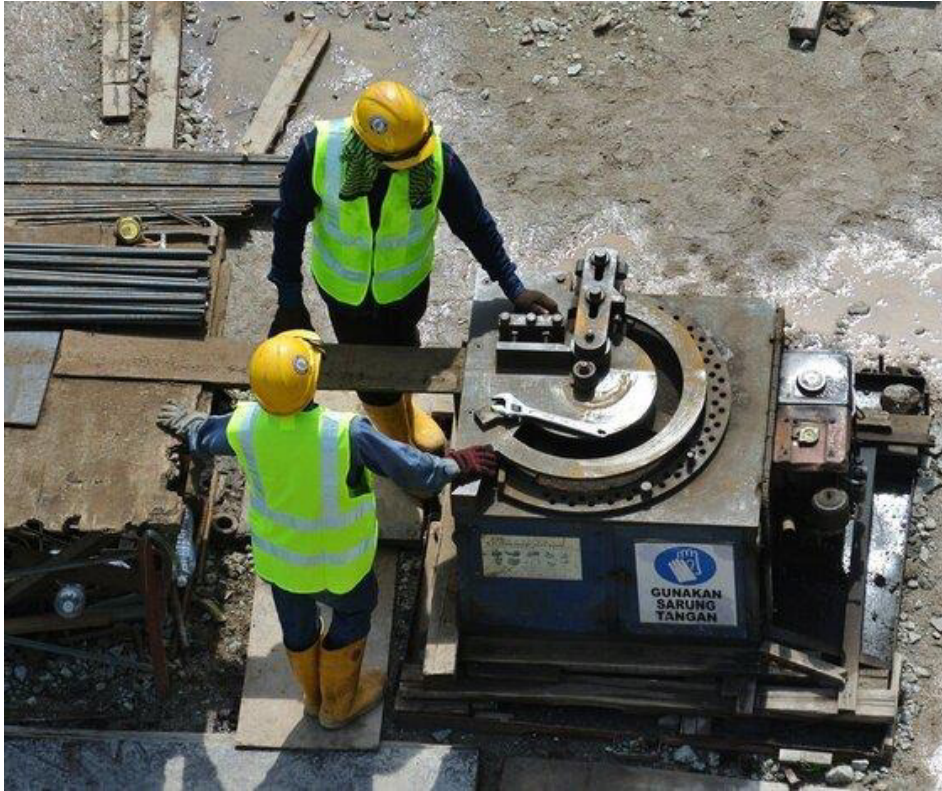
Fig. 4.4.3: Posture during bar bending/cutting
