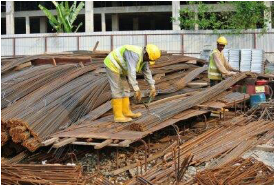
Fig. 4.4.12: Handling of rebars
