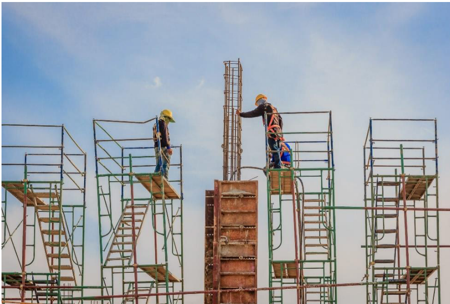
Fig. 7.1.4 Coordination during Construction Work
