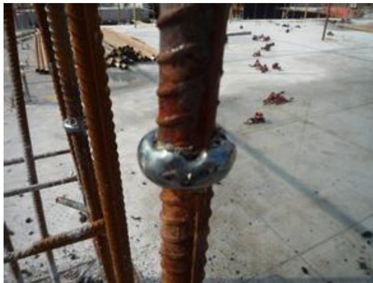
Fig. 5.1.8 Welded splicing
