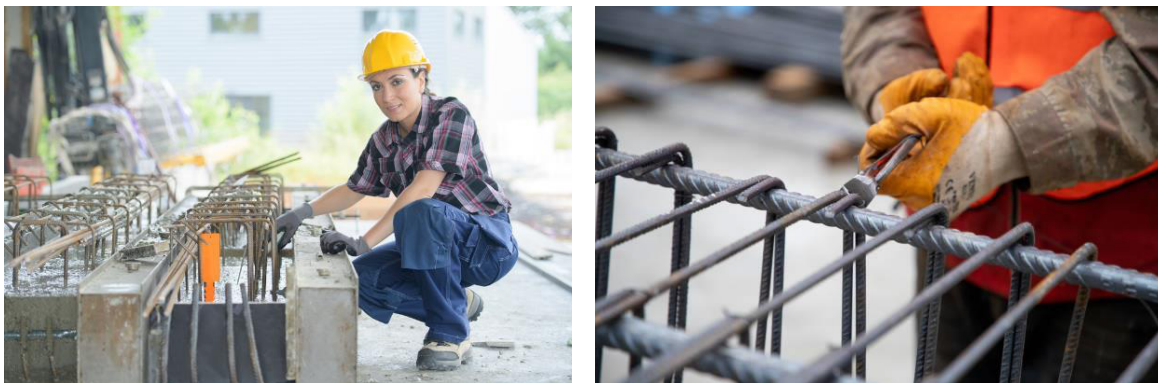
Fig. 1.2.2 Bar bender and steel fixer
