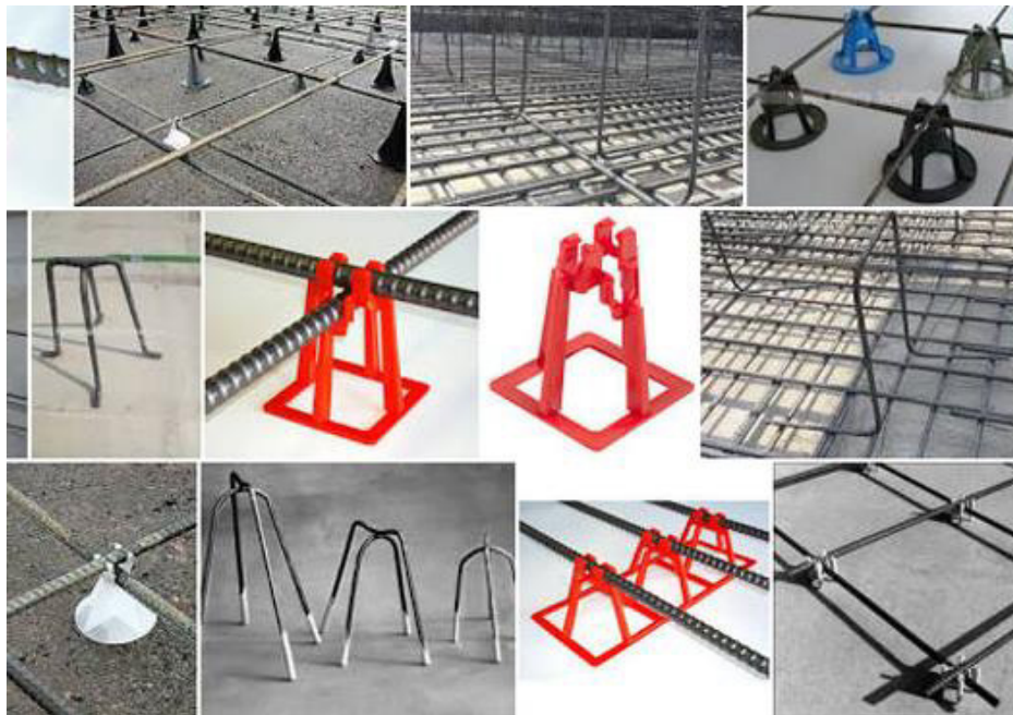
Fig. 4.2.22: Rebar spacers and chairs
