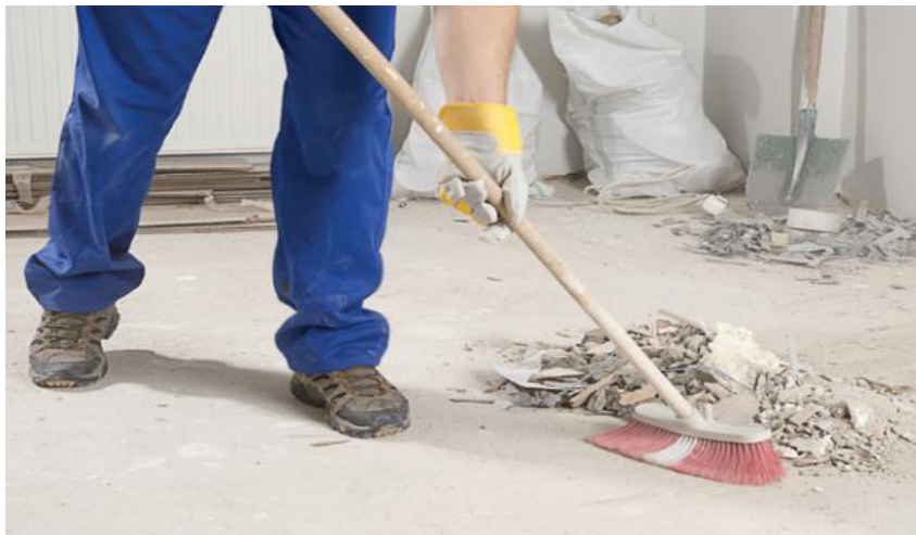
Fig. 9.3.5 Clean-up Debris and Waste
