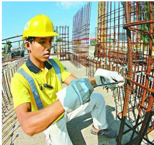
Fig. 1.2.3 Bar bender performing work at site
