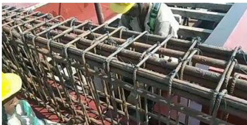
Fig. 5.3.4 Lapping of reinforcement bars
