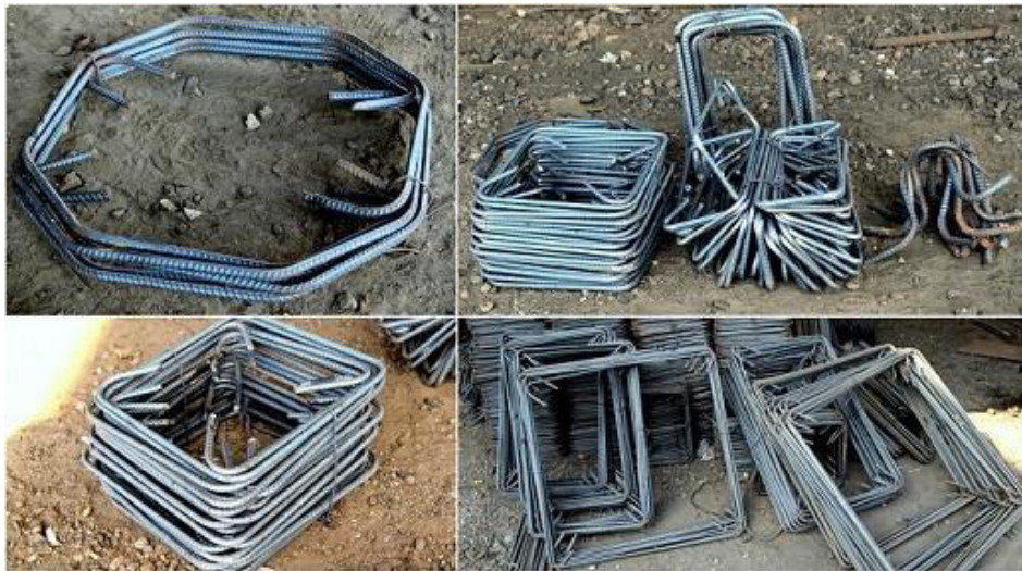
Fig. 5.3.5 Tagging and stacking of prepared reinforcement materials
