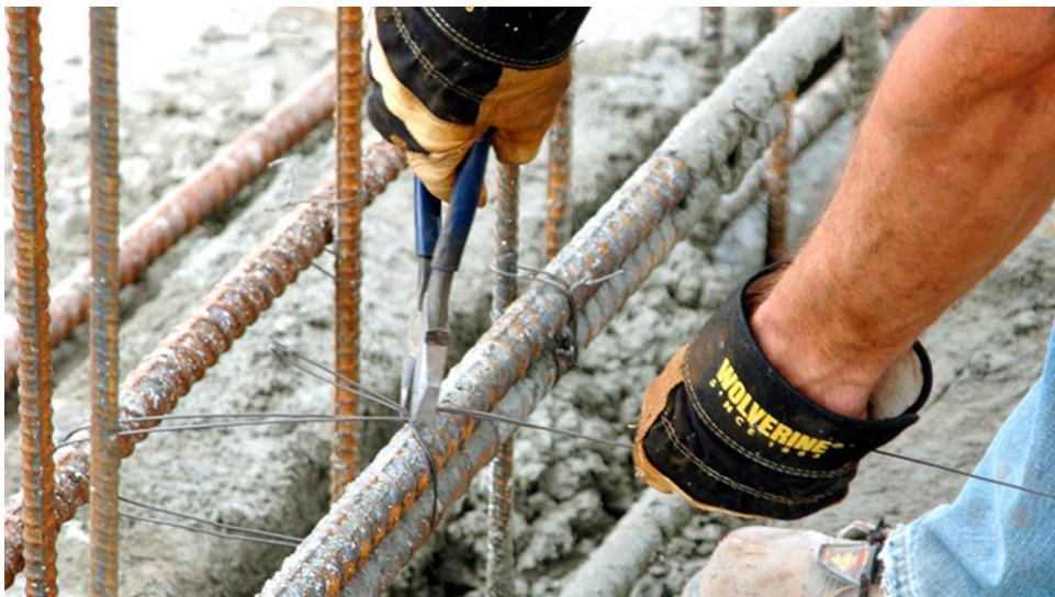
Fig. 5.1.2 Tying rebar (reinforcement bars) using wire
