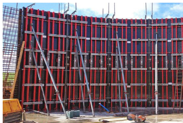
Fig. 1.1.14 System formwork
