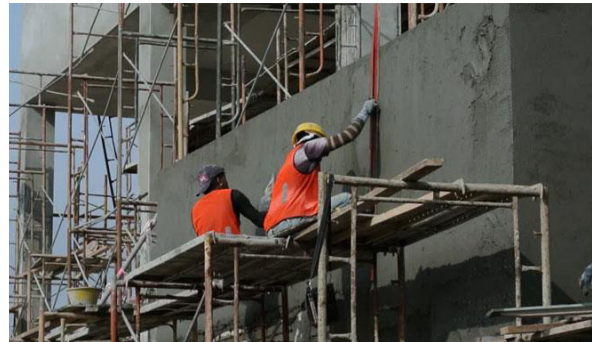
Fig. 1.1.10 Plastering Work
