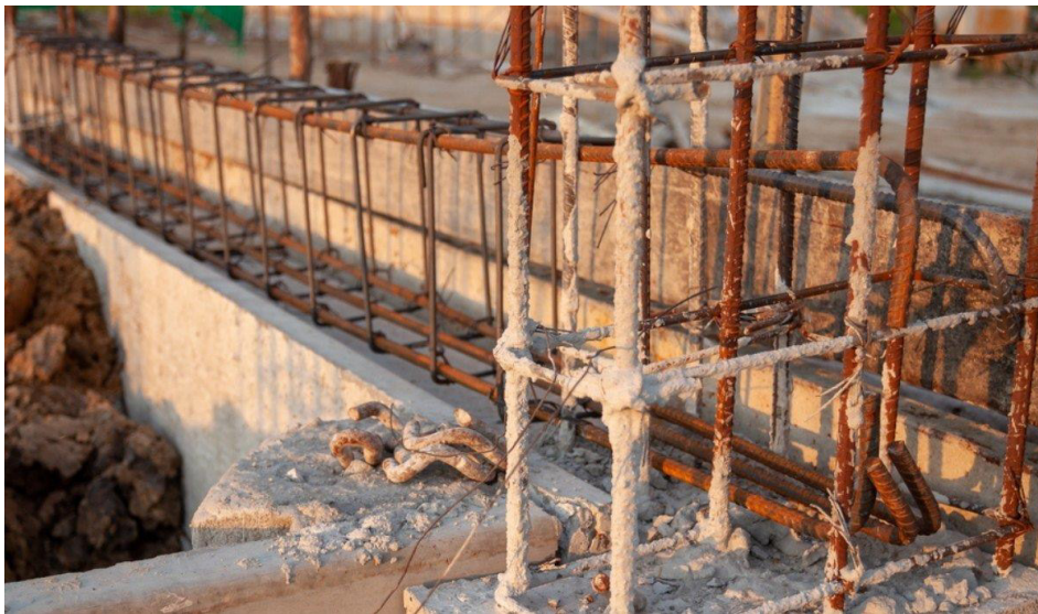
Fig. 6.2.2 Beam ties
