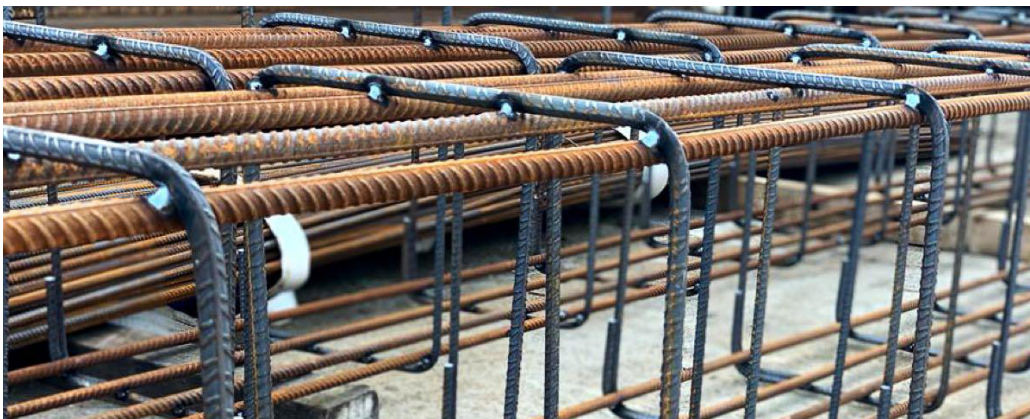
Fig. 5.3.7 Fabricating a steel cage
