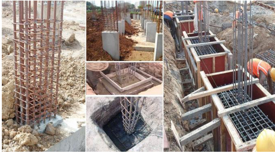
Fig. 6.3.3 Erecting temporary supports and marking layouts for various RCC structures
