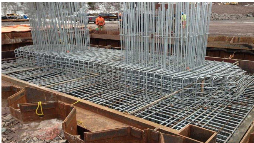
Fig. 5.2.5 RCC cage fabrication process
