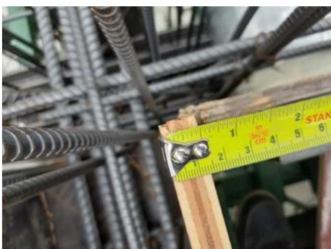
Fig. 1.2.4 Measuring of a rebar
